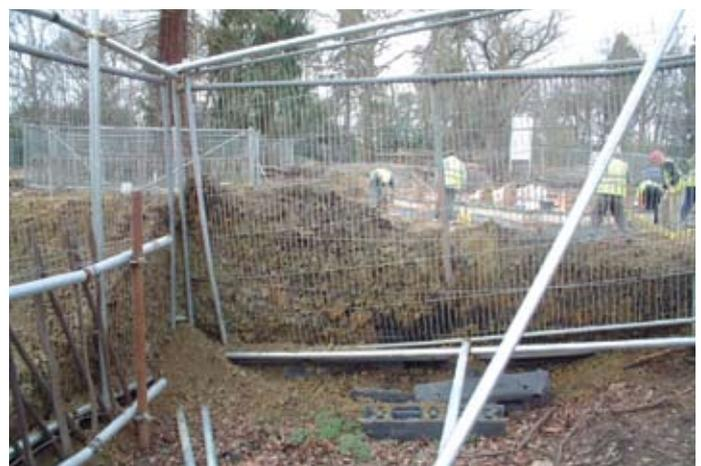
Braced fencing is important because it is difficult to imagine the pressures that have to be withstood when writing the specification in the comfort of the office!
