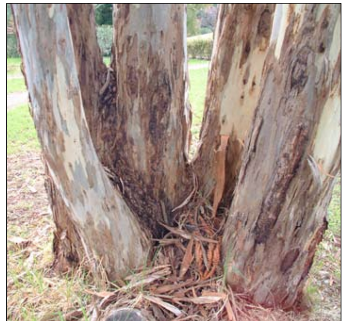
Z5-2: The base of the tree with the yellow box in photo Z5-1. Although the multiple stems could be considered defects, there are no obvious indications that there is a high risk of failure, which would make this tree an A2 and not Z5.
