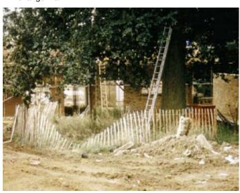
Paling fencing never has been effective at preventing encroachment and is not suitable for the modern development scenario.
